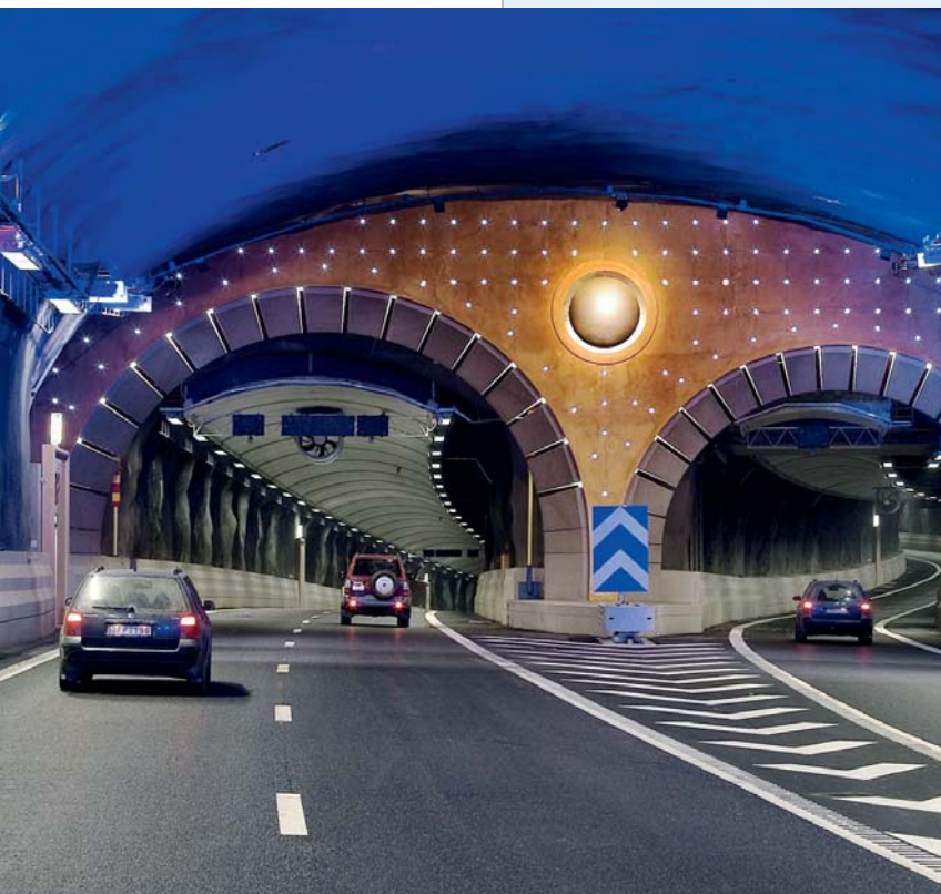
Tunnel with nano-coated guard rails on the side to reduce their tendency to soil and make them easier to clean
