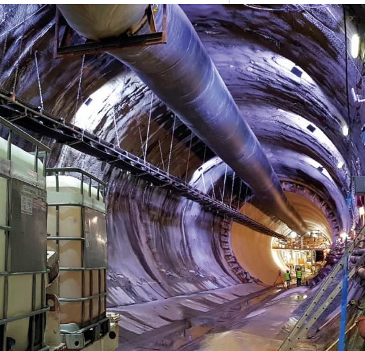
„Deep Tunnel Storm Water System“ in Dubai
