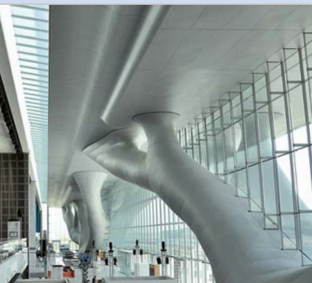
Qatar National Convention Centre, Doha
